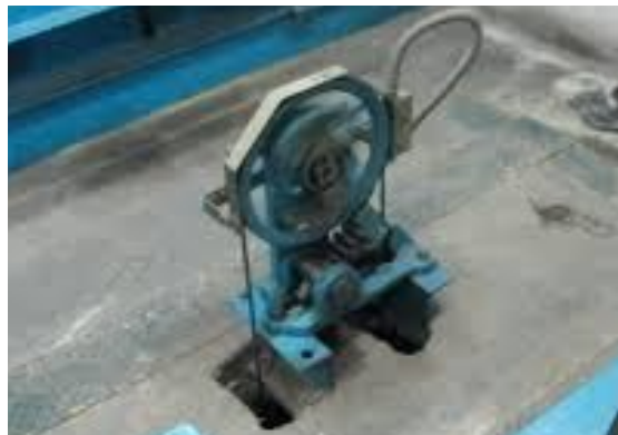
Diagram 6.17 Overspeed Governor in Elevator
