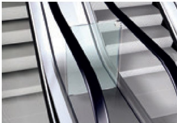
Diagram 6.31 Anti-Slide device installed to avoid sliding of objects or people
