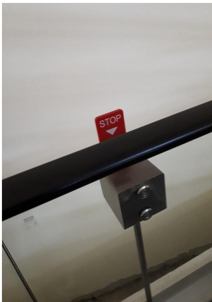
Diagram 6.33 Emergency Stop Device installed at the side of handrails to ease user triggering the brakes
