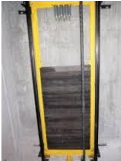
Diagram 6.14 Counterweight balancing the elevator and its load
