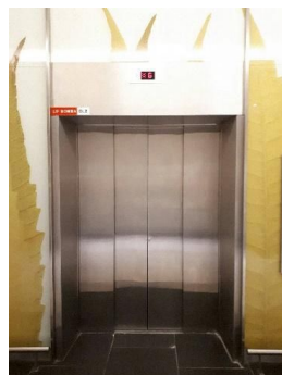
Diagram 6.5 The firefighting lifts in Summit USJ are labelled with red sign stating 'Lif Bomba'
