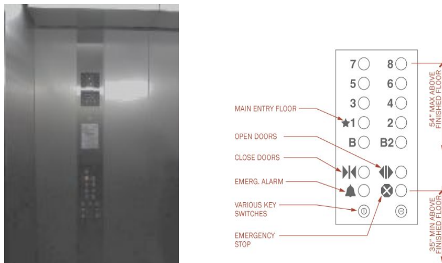
Diagram 6.10 Elevator at Summit (left) Illustration of the buttons and controls (right)
