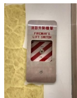
Diagram 6.4 The Fireman switch installed on the side façade of the elevator
