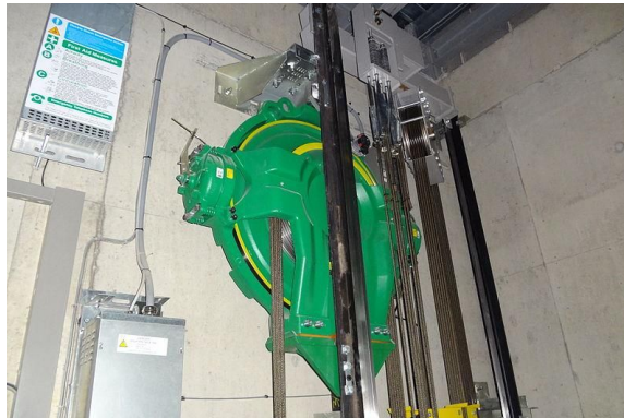
Diagram 6.10 Ecodisc Motor installed within hoistway
