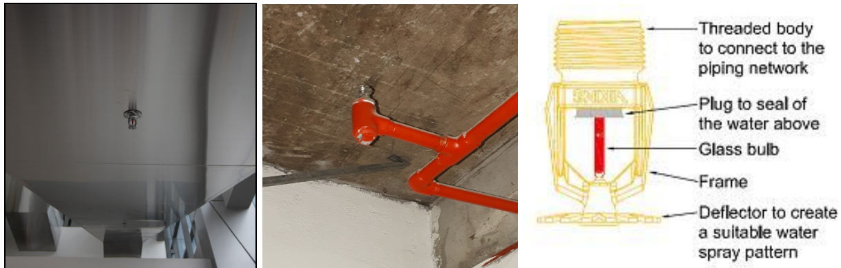
Diagram 5.22, 5.23 and 5.24 Pendant Sprinkler (Right), Upright Sprinkler (Middle), Components (Left)
