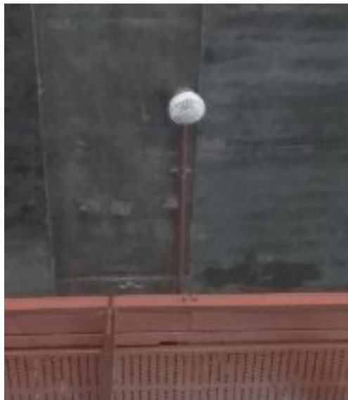
Diagram 5.3 Photoelectric smoke detector used in Summit USJ (Left), Detection process (Right)
