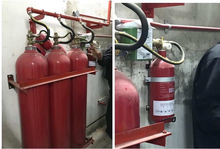
Diagram 5.18 and 5.19 Carbon dioxide tanks connected to the system
