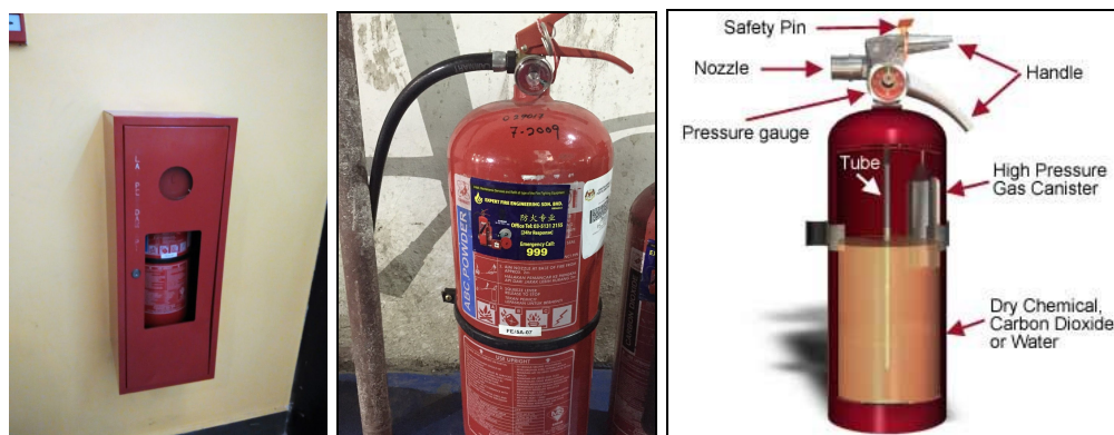
Diagram 5.15, 5.16 and 5.17 Container of extinguisher (Left), Extinguisher (Middle), Components of extinguisher (Right)
