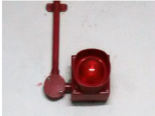
Diagram 5.9 Alarm bell with a siren light installed.
